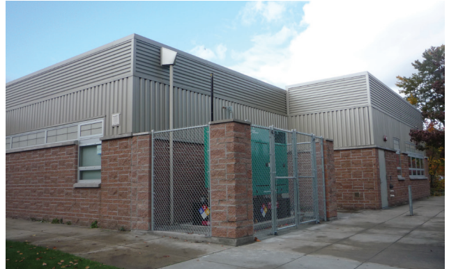
EDMONDS SD MEADOWDALE HS | GENERATOR REPLACEMENT
