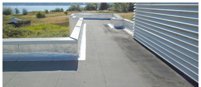
NOAA WRC | ROOF ASSESSMENT
