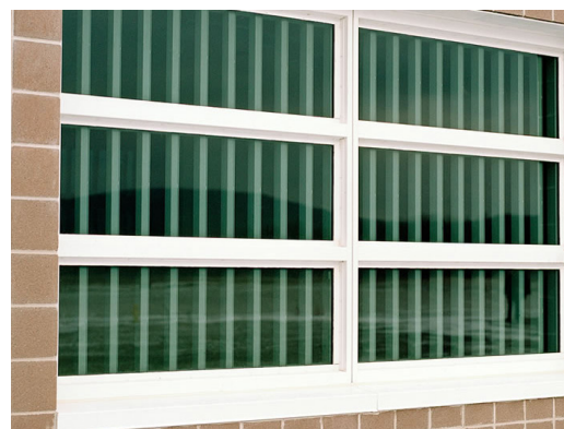
CORRECTIONAL FACILITY | WINDOW REPLACEMENTS
