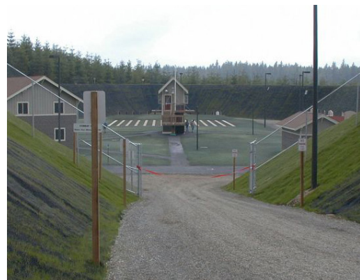
RAVENSDALE SHOOTING RANGE STRUCTURAL IMPROVEMENTS
