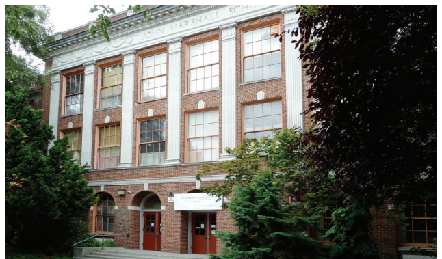
SPS JOHN MARSHALL SCHOOL | CONDITION ASSESSMENTS
