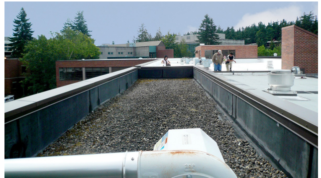
WWU FINE ARTS BUILDING | ROOF REPLACEMENT
