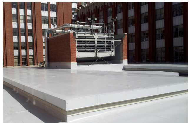
US GSA FEDERAL OFFICE BUILDING | ROOF REPLACEMENT
