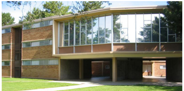
CWU STEPHENS-WHITNEY HALL | TENANT IMPROVEMENTS
