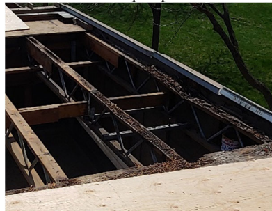
Decayed roof joist (requiring replacement)
