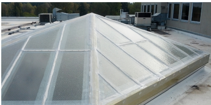
Skylight Replacements, Pierce College
