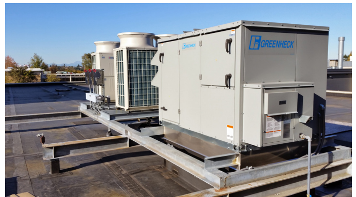
Mechanical Upgrades & Replacements, South Seattle College
