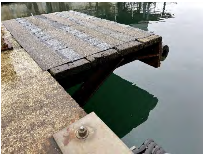
Photo 61: Balcony loading platform
