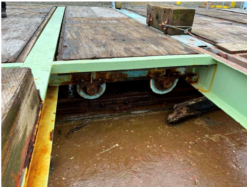
Photo 181: Cradle wheels and decking
