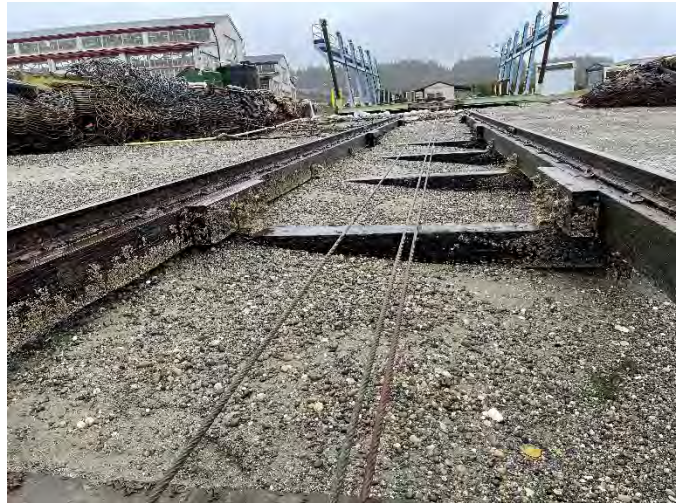
Photo 170: Rail system looking North
