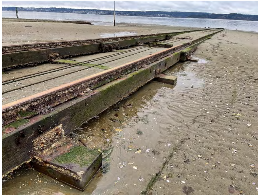
Photo 173: Rail system looking South
