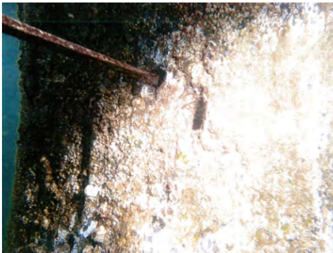
Photo 12: Pile 3B two marine borer entries (MBE)
