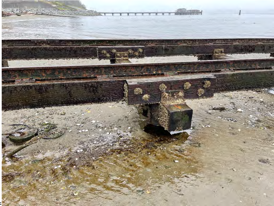
Photo 140: 11 th pile cap from bulkhead
