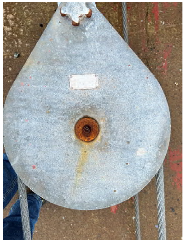
Photo 175: Snatch block on South end of cradle
