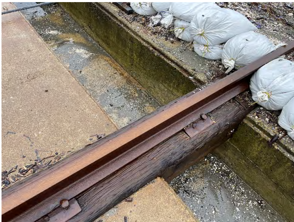
Photo 132: Timber rail and rail North of bulkhead
