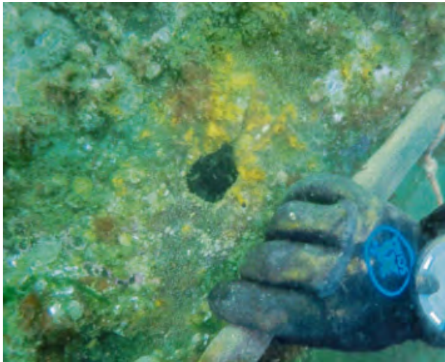
Photo 37: SP3-B holed through
