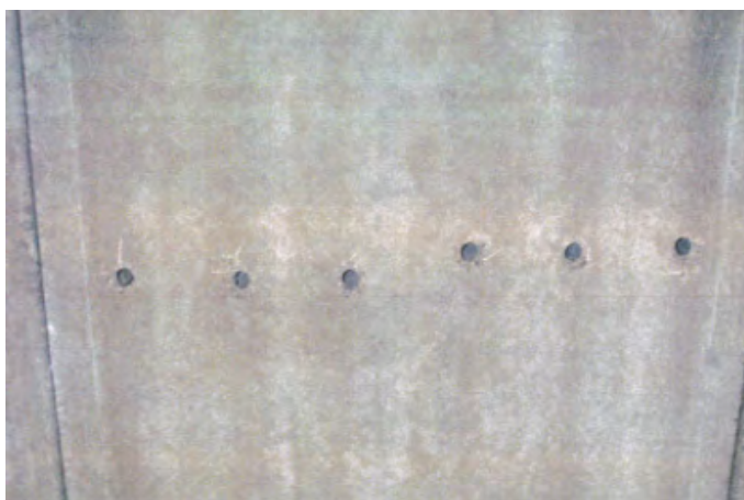
Photo 16: 1" diameter holes drilled at midspan of precast deck
