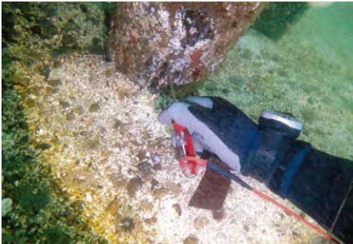
Photo 93: Right wingwall, pile 31 with MBE
