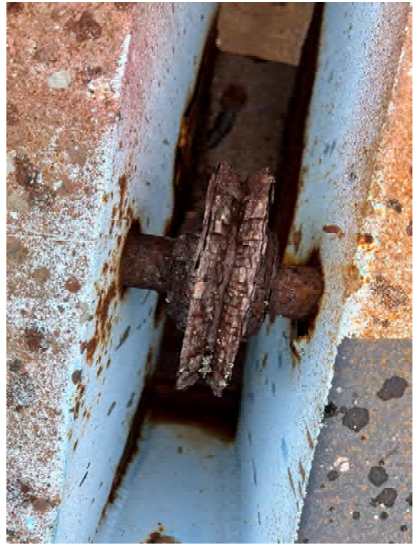
Photo 192: Bilge block pulley
