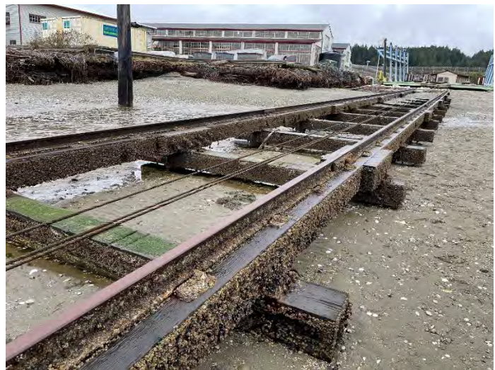
Photo 172: Rail system looking North
