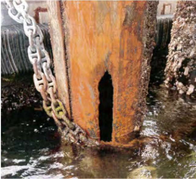
Photo 39: SP4-A holed through
